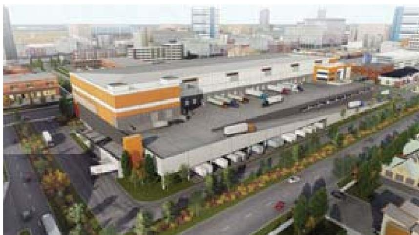
*Rendering by Ware Malcomb of a multi-story industrial building with a two-level truck court and multiple two-way ramps to enable multitenant occupancy. (From NAIOP)*
